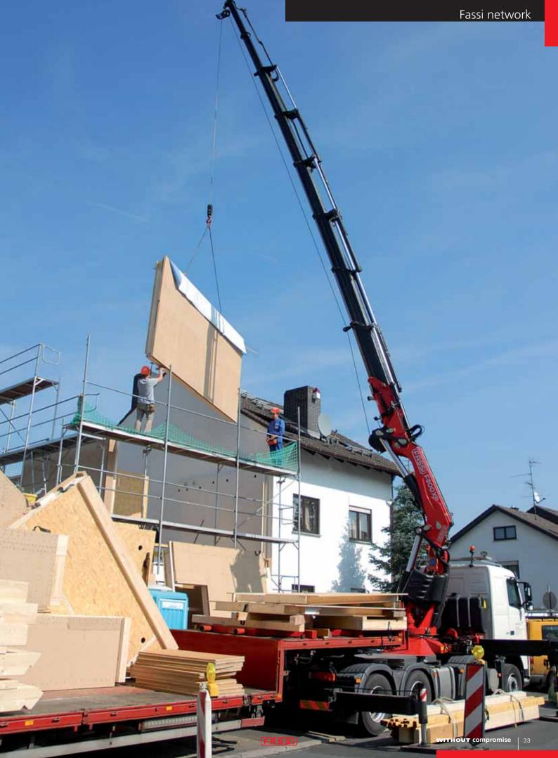
2505 kg) and is equipped with an additional boom (jib) giving a total extension of up to 32.20 m (lifting capacity 270 kg).
