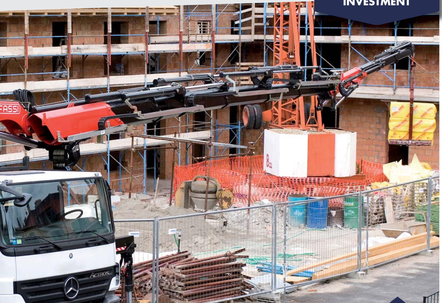
The F660RA crane in action. It's a heavy-duty crane and it lift up to 60tm
